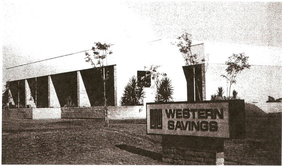
1974 Tempe Mall Branch, 1801 E Southern Avenue. John W. Dick, architect. (Courtesy of architect)
