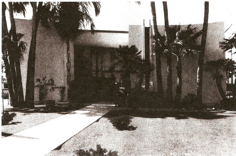
1965 Yuma Branch, 1690 S Fourth Avenue. Bennie M. Gonzales, architect; remodelled by Brock & Craig, 1982. (A. M. Hammer)
