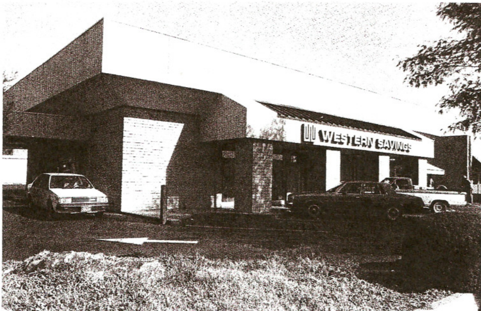
1960 East Thomas Branch, 3800 E Thomas Road, Phoenix. Calvin M. Butler, architect. (A. M. Hammer)
