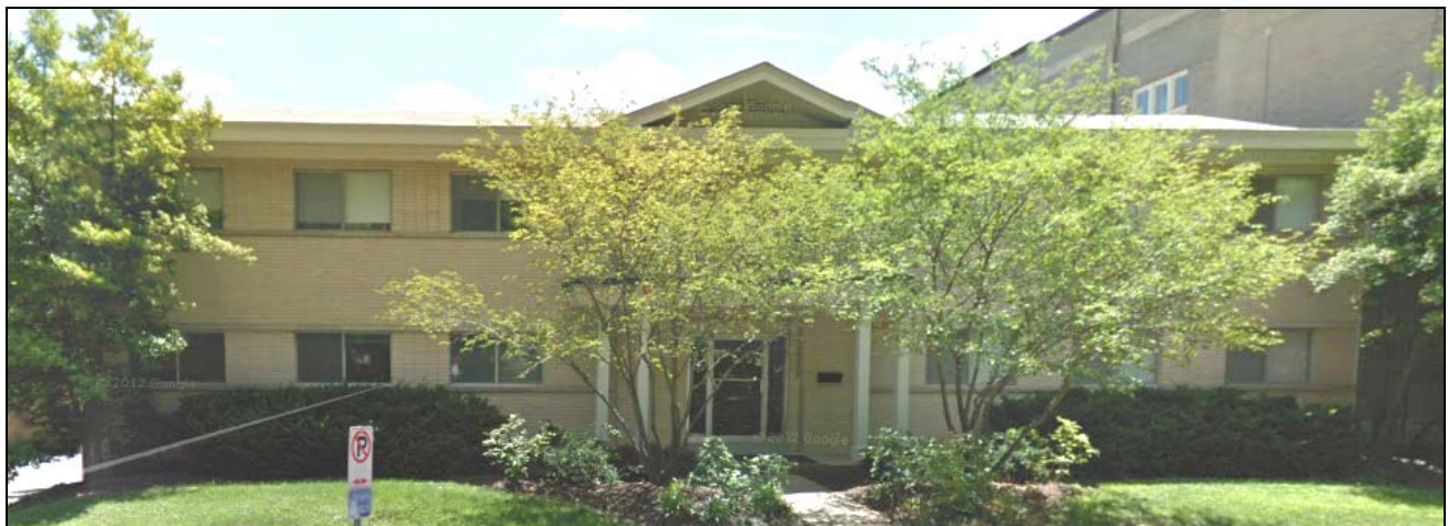
FRONT ELEVATION OF RESIDENCE
