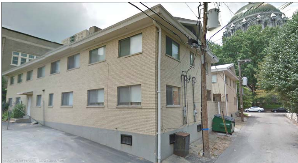
REAR AND NORTH ELEVATION
