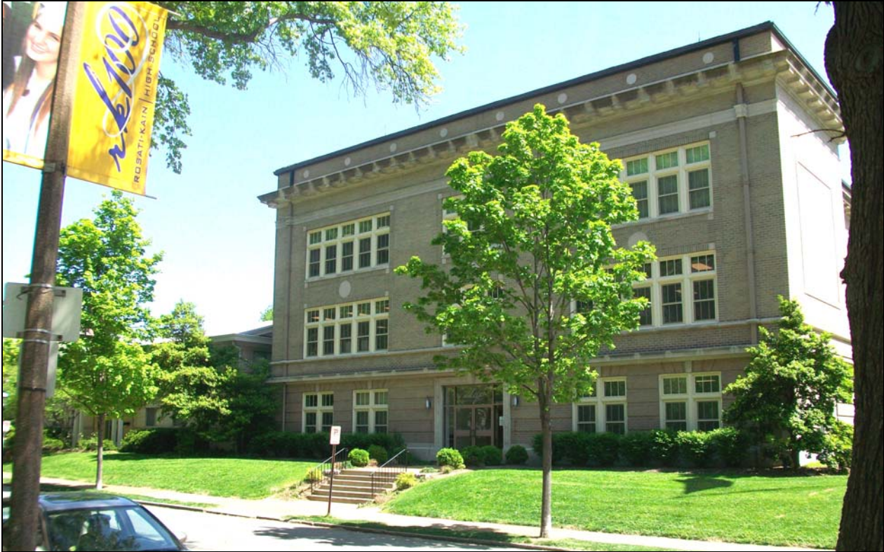
EXISTING WEST FAÇADE OF ROSATI-KAIN WITH NUNS' RESIDENCE IN SHADE AT LEFT
