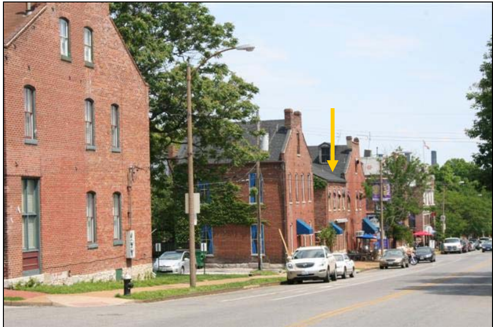
ROOF AS SEEN FROM WEST AT CORNER OF RUSSELL AND 11 th
