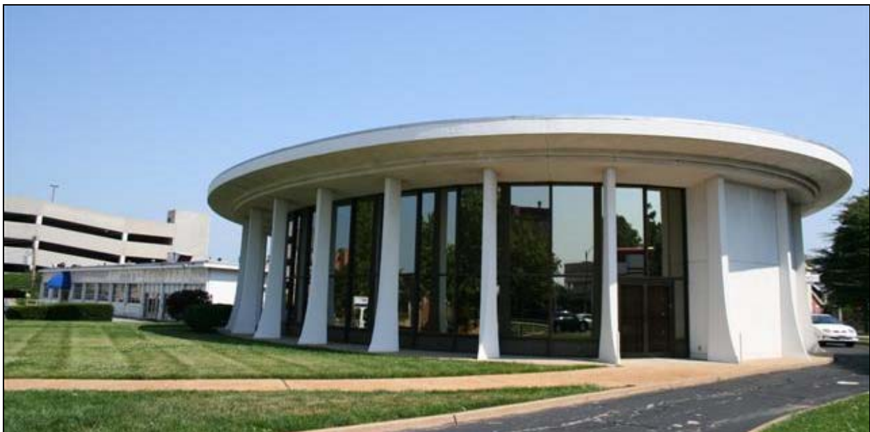
AAA BUILDING LOOKING NORTHWEST WITH GARAGE BUILDING IN BACKGROUND
