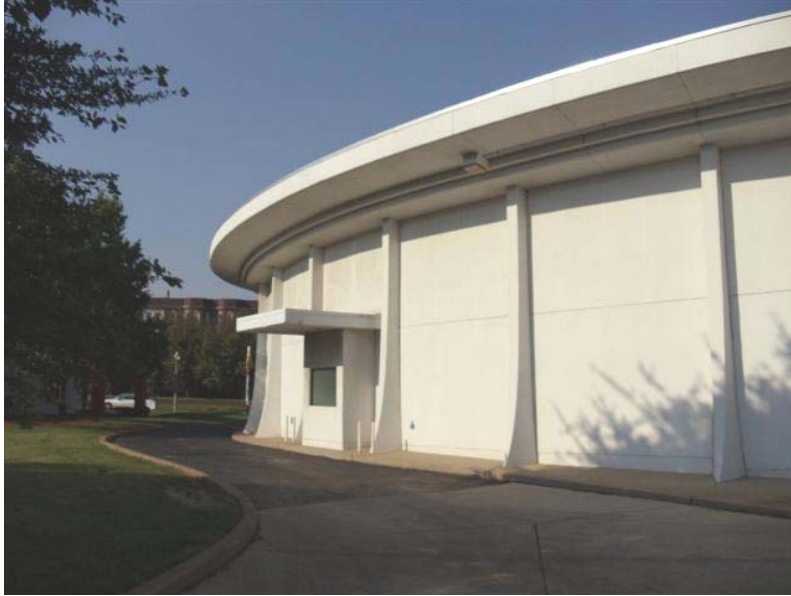
DRIVE-UP WINDOW ON McPHERSON SIDE OF BUILDING
