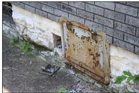
COAL CHUTE IN LIMESTONE FOUNDATION
